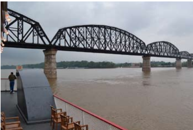
Big Four Bridge
